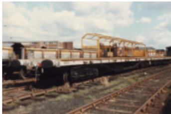
YMA Salmon DB996931 at Willesden in March 1987. This picture shows four types of Salmon. To the right is a YMA with curb rails, while on the track behind are two YFAs with rail cranes, one with canopy and one without.
